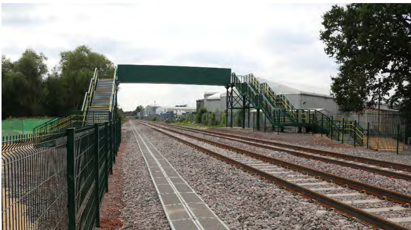
The first section of track to be commissioned near Bicester Fringe
